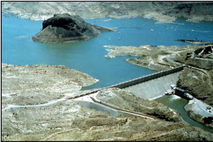
Elephant Butte Dam. Photo Source: U.S. Bureau of Reclamation
